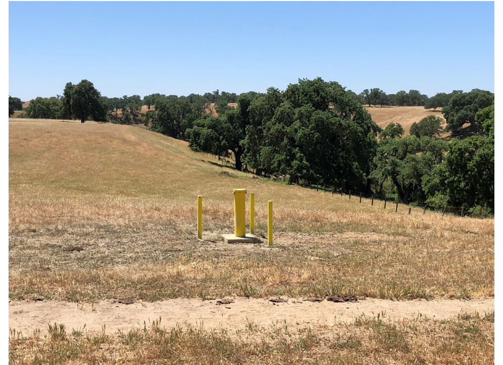
Representative Monitoring Well MW-9
